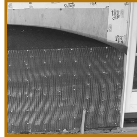
Application of galvanized lath to exterior wall.
