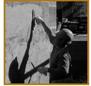
Application of scratch coat to surface of exterior wall.
