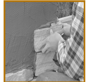
Application of Natural Thinstone Veneer.
