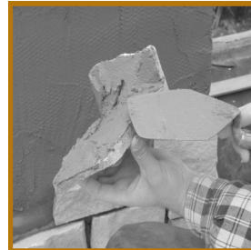
Application of mortar onto Natural Thinstone Veneer.
